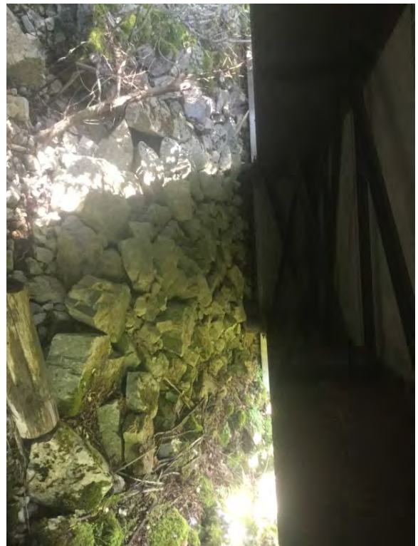
Right Bank Abutment when facing downstream
