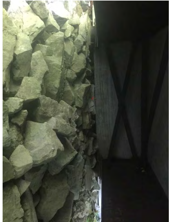
Left Bank Abutment when facing downstream
